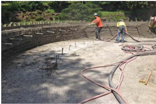
Fig. 6: Shotcrete placement at Royal Botanical Gardens Rock Garden pool
