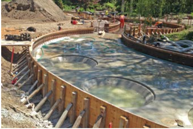
Fig. 5: Single-sided formwork at Royal Botanical Gardens Rock Garden pool, Hamilton, ON, Canada
