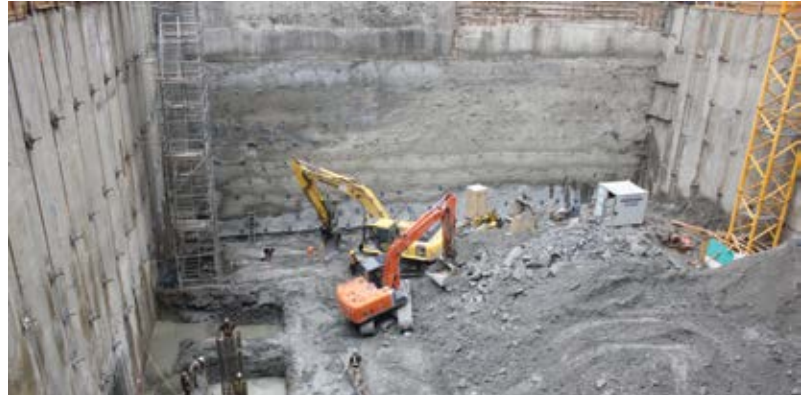
Fig. 3: Excavation in progress on the east elevation
